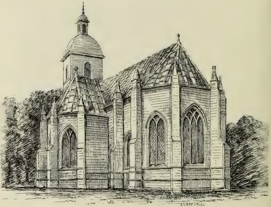
FIG. 1143.—Ladykirk Church. View from South-East.
